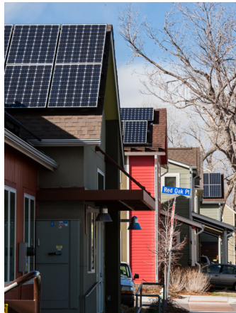
Shading can greatly affect power output. Examine effects of seasonal sun angles, new buildings and growing trees.
