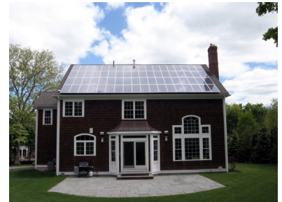
Roof-mounted solar array for large power capacity.
