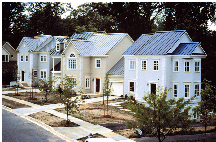
Flexible thin film solar panels blend in between the ridges of metal roofing.
